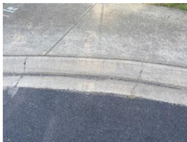
Figure 3. Cracked curb on Pound Street (12/12/2023)
