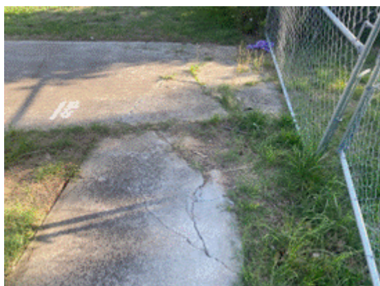
Figure 4. Damage to council footpath near driveway (12/12/2023)
