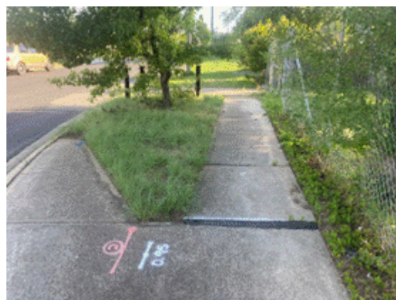
Figure 5. Roots lifting foot path on Pound Street (12/12/2023)
